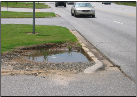
Damage due to insufficient curb radius
