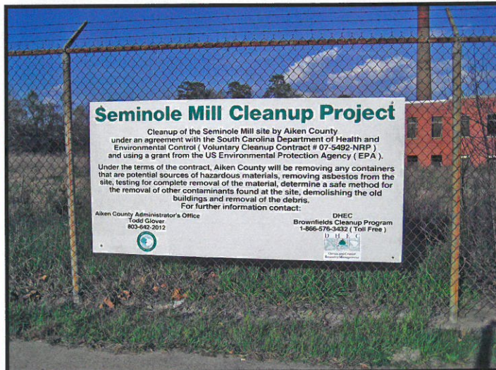
Seminole Mill in Aiken County undergoing demolition and cleanup
