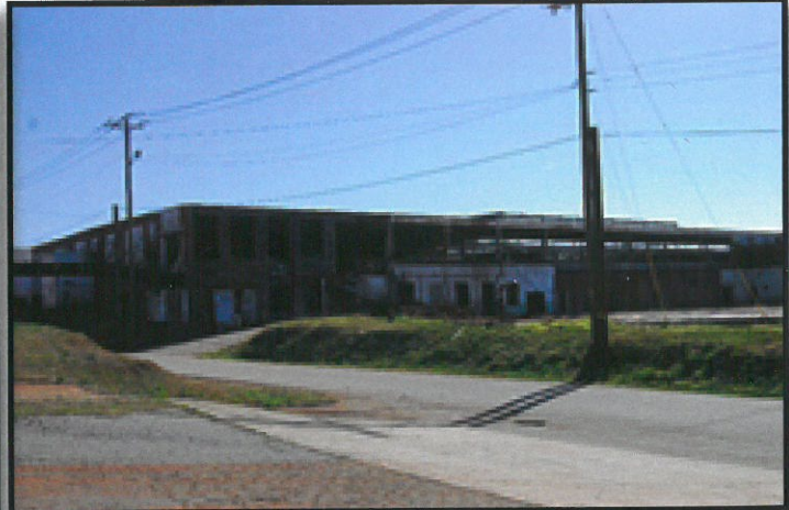
Abandoned Piedmont Shirt Factory in Greenville County before demolition and soil cleanup by Greenville County Redevelopment Authority
