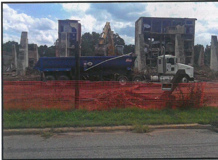
Demolition and cleanup of Victor Mills in Spartanburg County
